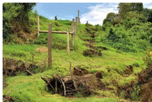
A completed section of the fence being constructed around the forest
